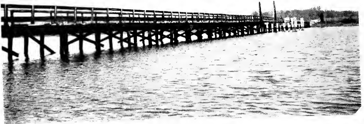
OLD WYE ISLAND BRIDGE
